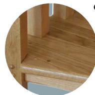
We finish the process by providing nosing on all the outer edges of the treads corners for a professional look. With all the extra effort and detail, the finished solid wood treads are a thing of beauty.
