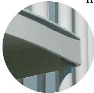
Take a closer look and you'll see all the welds are hidden on the underside of the treads to create crisp looking lines. To further enhance the beauty of the stair, all hub set screws are hidden between the tread supports (*on continuous sleeve treads*). Set screws lock the hubs to the inner column and stabilize the treads around the column. The result is a strong center column free of visible set screw holes.
